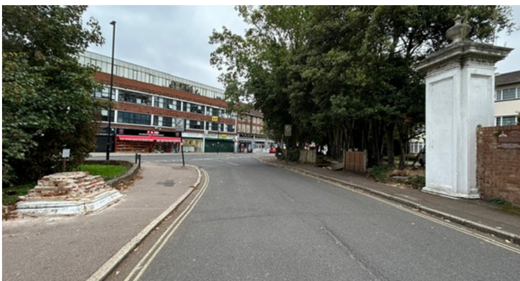
Canons gate piers showing the remains of the damaged pier on the left hand side of the picture.
